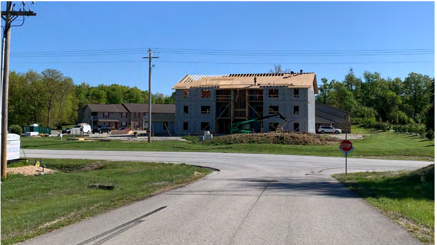
Multi-family housing construction at the corner of SR 1 and SR 46 near the interchange. Source: HWC Engineering
