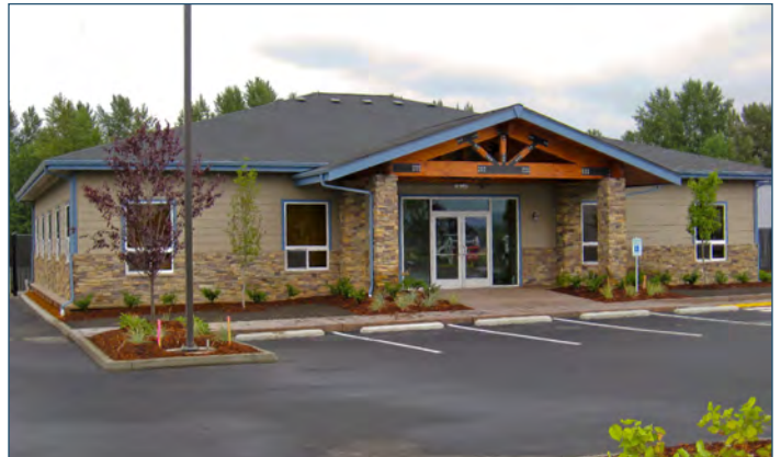
An example of a small, freestanding office building that would be appropriate for the SR 1 area. Source: Pacific Mobile Structures, Inc
