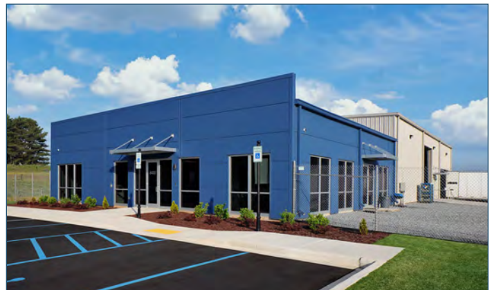
Rural manufacturing building. Source: Shutterstock
