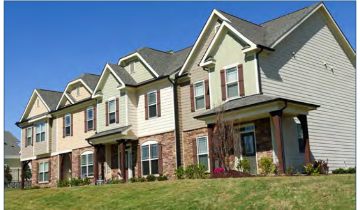
Townhomes introduce multi-family units while respecting surrounding community character. Source: Home Advisor
