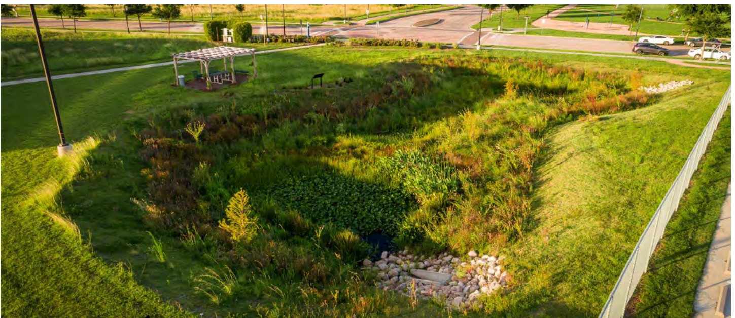
Future development should include stormwater management infrastructure to slow runoff volumes and increase infiltration. Source: Bryan Malloch
